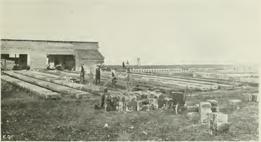
FIG. 21.—BLOCKS LAID OUT FOR SEASONING, CRAYFORD.
